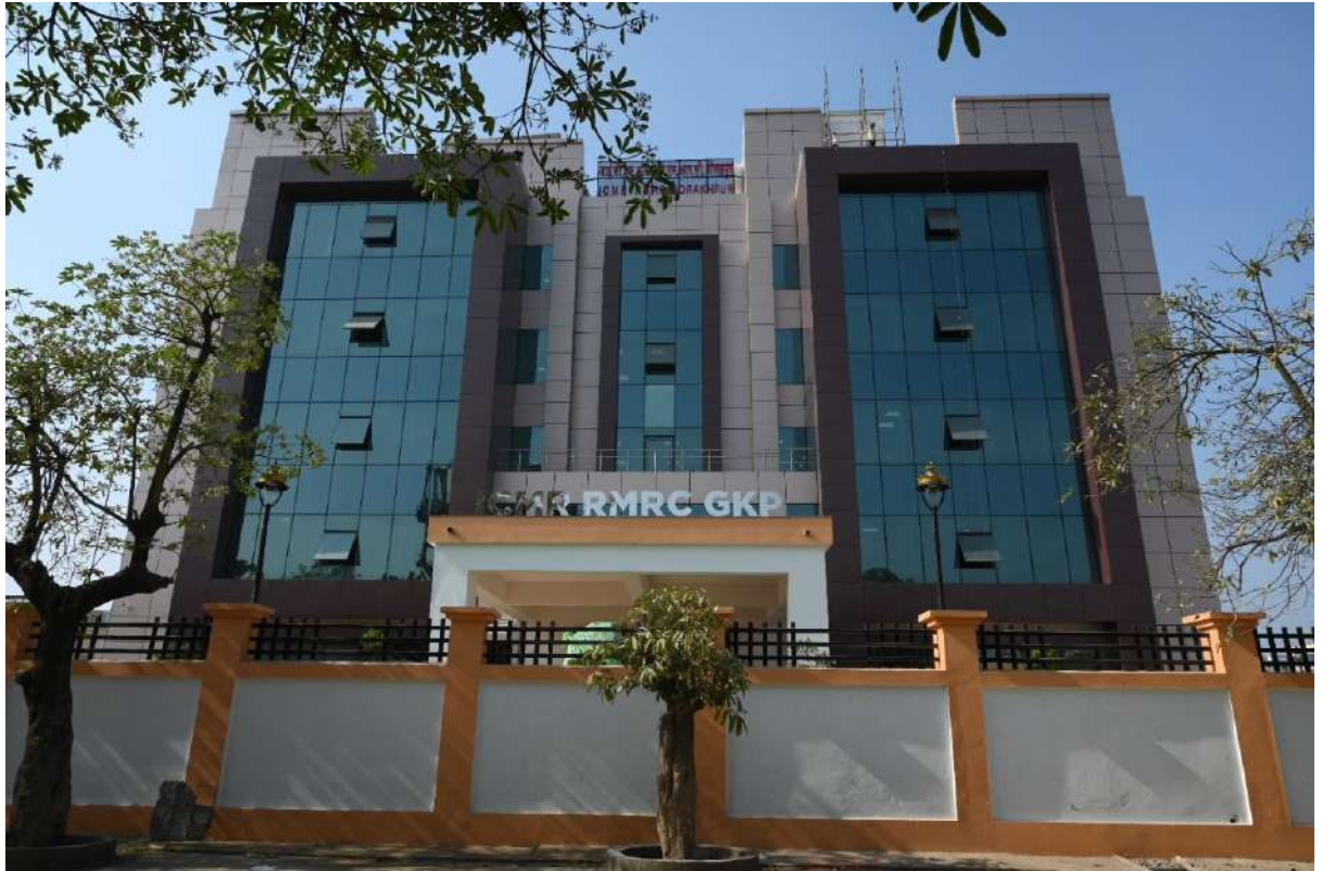
New building of ICMR-RMRC Gorakhpur
